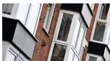
Figure 16 AIB exterior painted panel
