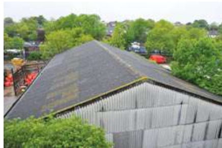
Figure 32 Asbestos cement roof and cladding
