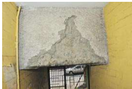
Figure 8 Sprayed coating on building passageway
