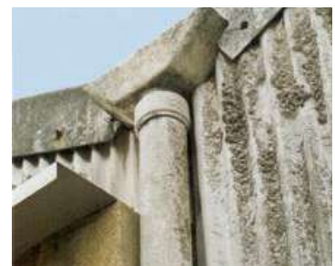
Figure 35 Asbestos cement downpipe
