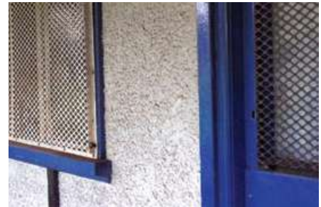
Figure 33 Chrysotile pebble-dash exterior wall coating
