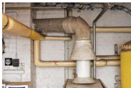
Figure 34 Asbestos cement boiler flue
