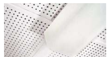
Figure 17 AIB ceiling tiles
