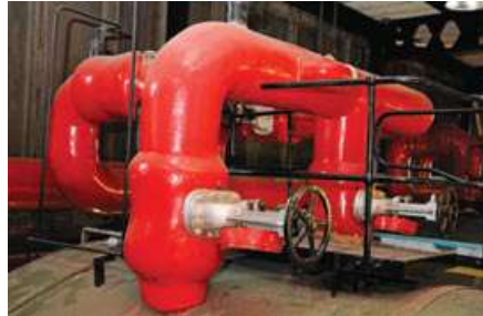
Figure 48 Asbestos-insulated supply pipes
