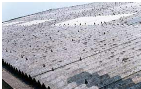
Figure 2 Asbestos cement: Work with this material does not require a licence
